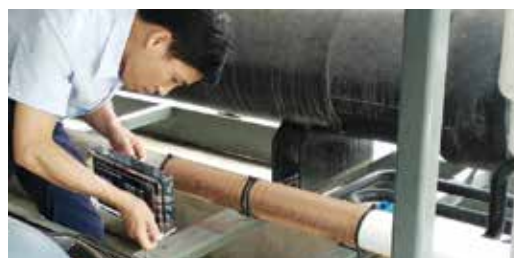
Installation de Vulcan S100
