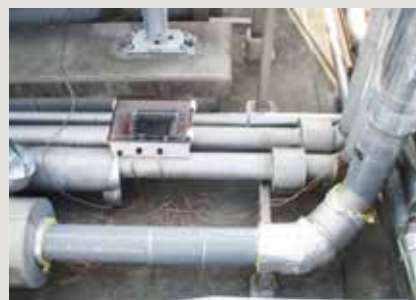
Installation de Vulcan S100
